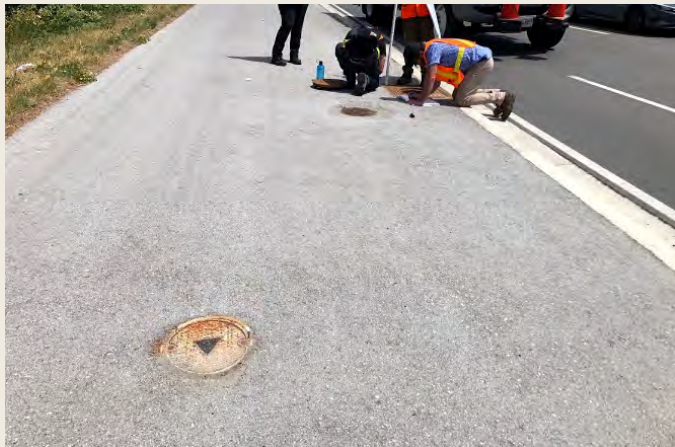
Figure: (Photo Left) Region of Peel and CVC staff conducting acceptance inspections of infiltration galleries along Queen St West in Brampton, ON; (Photo Right) Catch basin with snout protecting infiltration feeder pipe filled with sediment.
