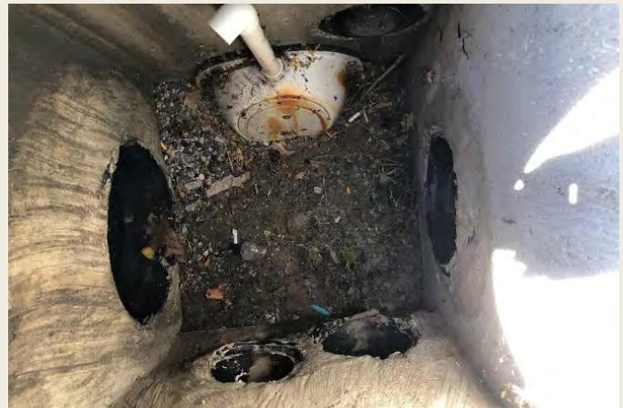
Figure: (Photo Left) Region of Peel and CVC staff conducting acceptance inspections of infiltration galleries along Queen St West in Brampton, ON; (Photo Right) Catch basin with snout protecting infiltration feeder pipe filled with sediment.
