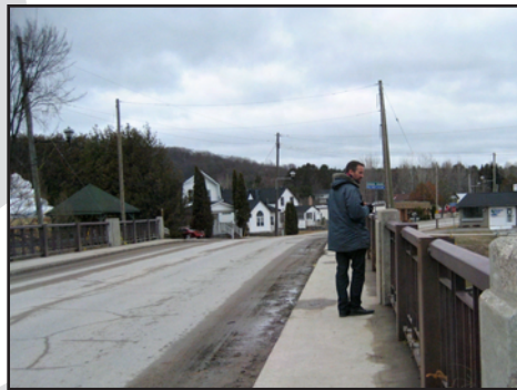
Narrow and cracked sidewalks over Gull River
