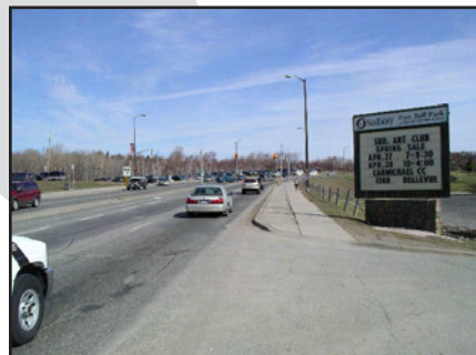
Entrance to Bell Park: Challenging for pedestrian access
