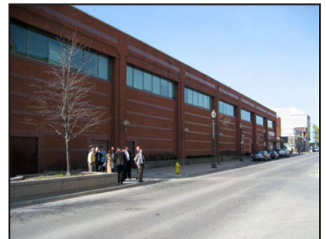
Inactive street frontage uninviting to pedestrians
