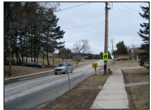
Incomplete sidewalks in school zone
