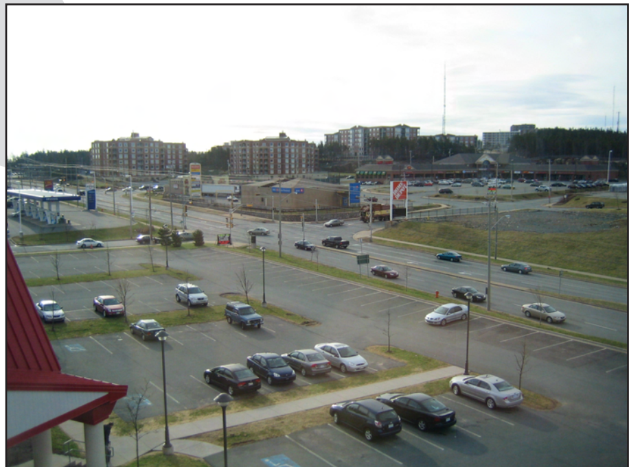
Bird's eye view of car-dominated Clayton Park big box development
