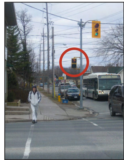
Poor systems result in non-compliance
