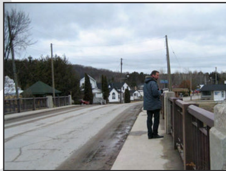
Narrow and cracked sidewalks over Gull River
