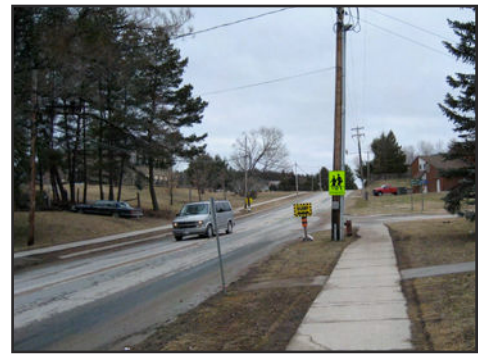
Incomplete sidewalks in school zone
