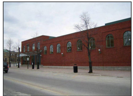
A blank wall facing the street creates dead space that is unwelcoming to pedestrians and can encourage crime
