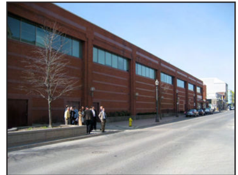
Inactive street frontage uninviting to pedestrians
